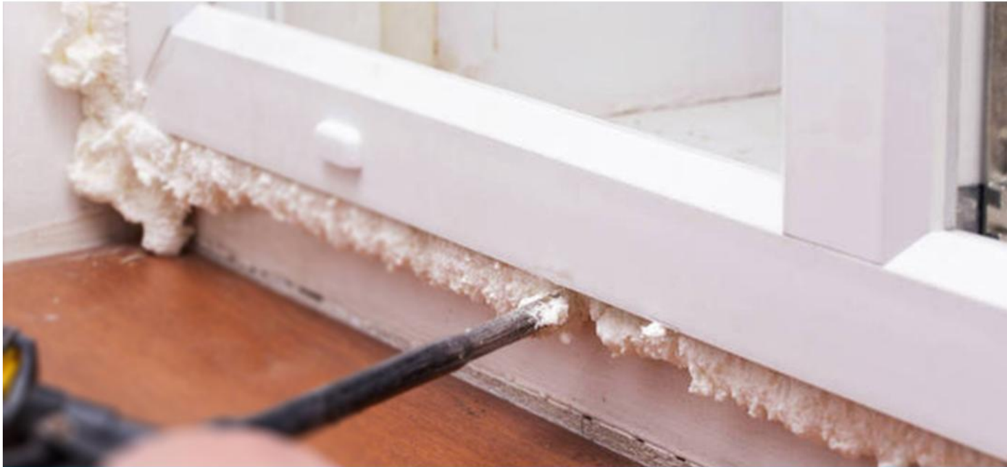
Installation of door and window frames
