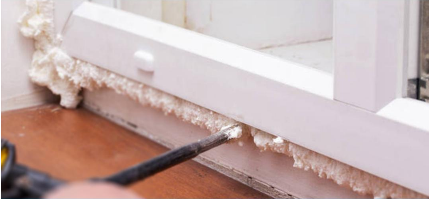
Installation of door and window frames
