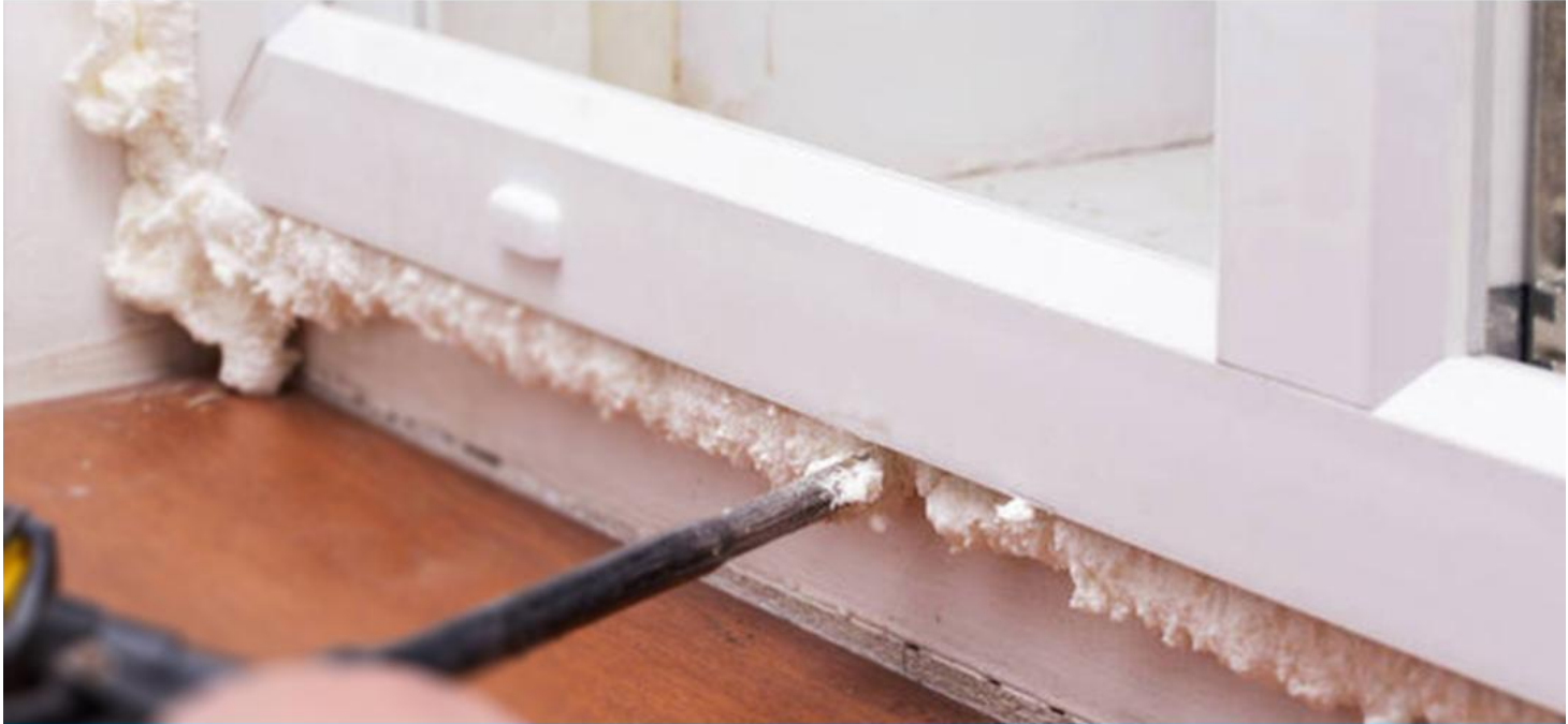
Installation of door and window frames
