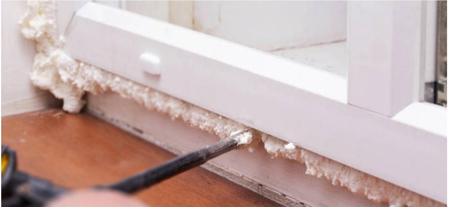
Installation of door and window frames
