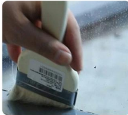
5. Remove Dirt, Grease, Moisture and Old Caulk
