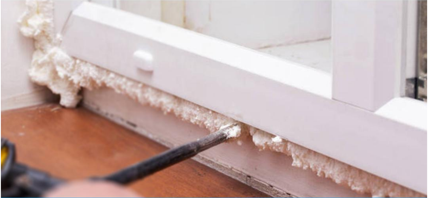
Installation of door and window frames
