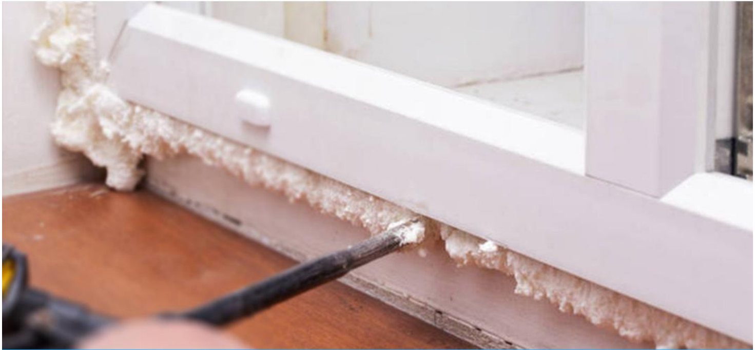
Installation of door and window frames
