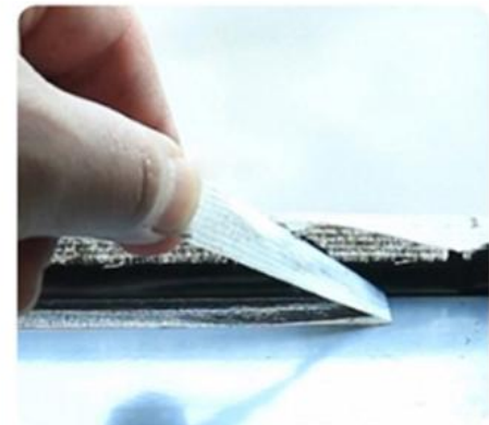
9.Remove Masking Tape Immediately
