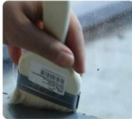
5.Remove Dirt, Grease, Moisture and Old Caulk
